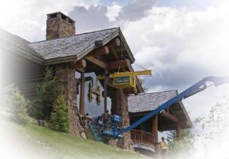
The CB2DCS Counterbalance Lifter was developed by Wood's Powr-Grip for use with a crane or other hoisting equipment, to lift and position windows under gables, overhangs or similar obstructions, by extending the load away from lift slings. This lifter's unique design features a DC-powered counterbalance, which moves on demand along a rugged I-beam to keep the lifter balanced, whether loaded or unloaded.
