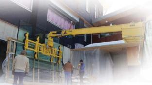
Wood's Powr-Grip® has created a new counter-balancer that is capable of lifting up to 2800 lbs. [1270 kg]. Redesigned with material and operator safety in mind, the CB3DCS counter-balancer functions in combination with the powerful MR16 vacuum lifter. For upper story window or curtain wall installation under an overhang, the CB3DCS is the ideal tool for the job.
